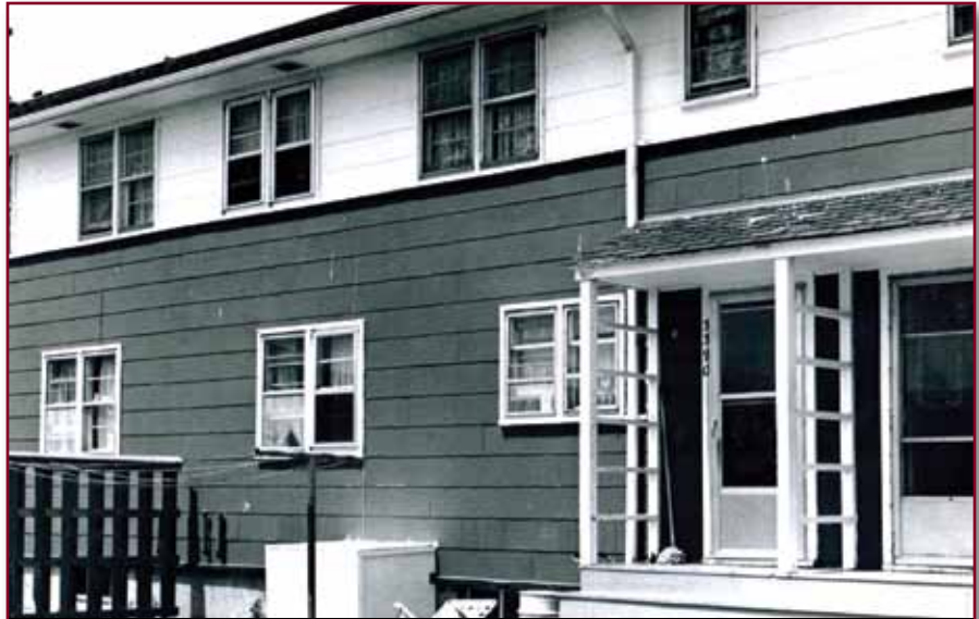
The rear of 3390 Federal Avenue, where the rescue took place. Landry climbed the white trellis onto the overhanging porch roof. He then shimmied across the gutter, broke the window with his helmet and swung up into the bedroom, which is to the left of the porch roof in the photo. July 13 1979. This shows the residence after it was restored and renovated.
